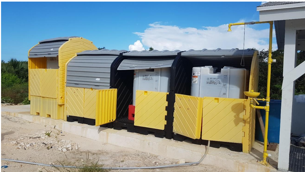
Figure 2.5 Sulphuric Acid Storage at Bogue WTP
